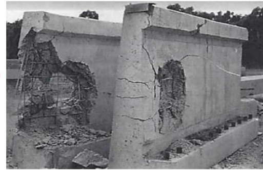
Fig. 2 Reinforced concrete wall targets (Walters, 1989)
