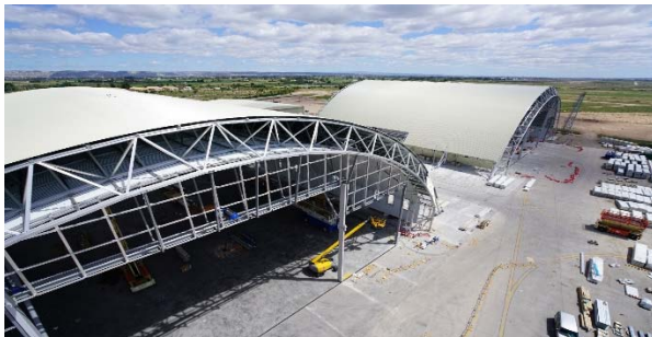
HANGARS - Zaragoza military airbase, Spain
