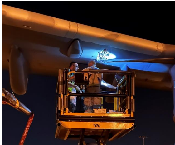
German CS performs maintenance on a fuel leakage on ES A400M
