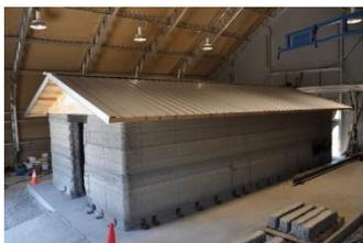
The US Army Construction Engineering Research Laboratory (CERL) successfully printed a 50 m<sup>2</sup> concrete structure, thanks to an AM technology called “Automated Construction of Expeditionary Structures” (ACES) aimed at printing semi-permanent structures in the field of operations. CERL is currently working with NASA to design, build, and test a third-generation concrete.
